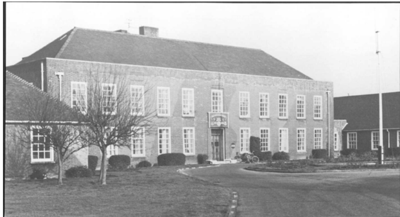
Building used by No. 3 Group
